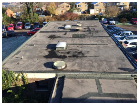
Maternity Lower Roof
