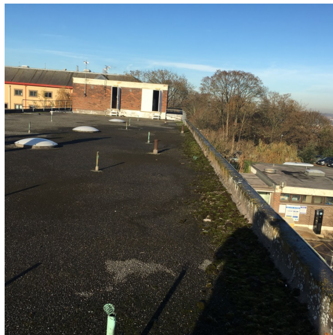
Maternity Roof and Roof Lights
