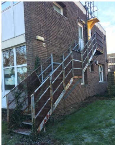
Maternity external fire escape
