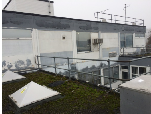
Oxford Building Cladding
